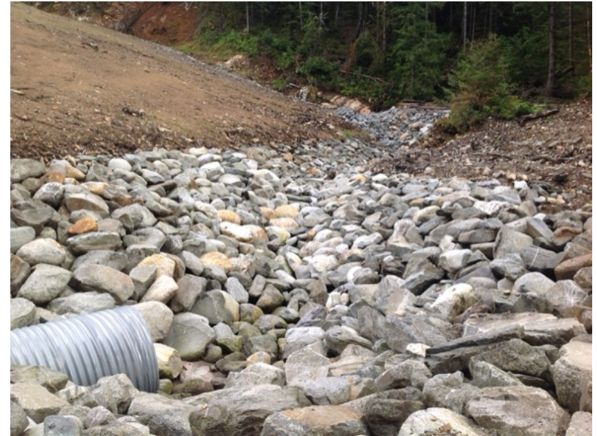
looking upstream from road surface
