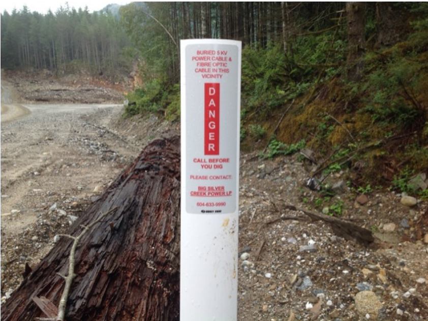
fibre optics line buried in road
